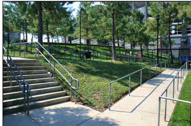
This wheelchair ramp at the Carolina Panther's stadium also benefits other users like bicyclists and parents with baby strollers.
