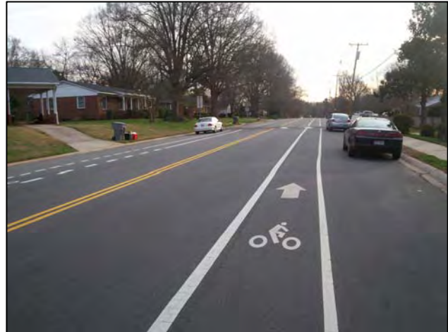
Careful placement of bike lanes away from the door zone adjacent to on-street parking is required
