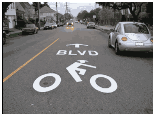
Pavement markers remind both bicyclists and motorists that the street is a Bicycle Boulevard
