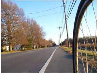
This photo was taken on 115 just south of Mount Mourne. This shoulder is approximately 3 feet wide, but a minimum of 5 feet is preferred.
