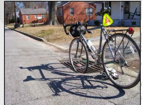
Roadways have hazards to bicycles.
