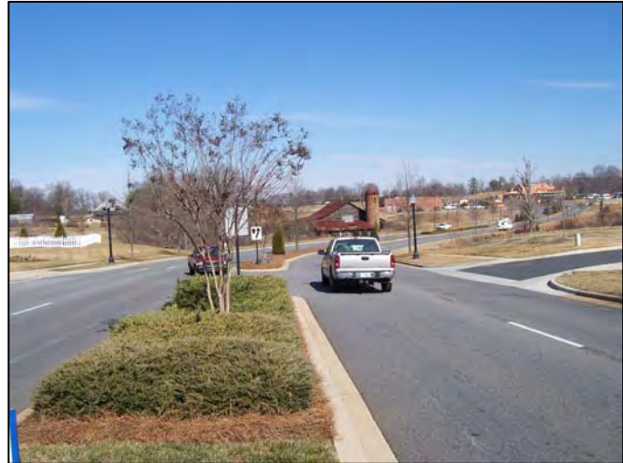
Morrison Plantation's four-laned residential roadway
