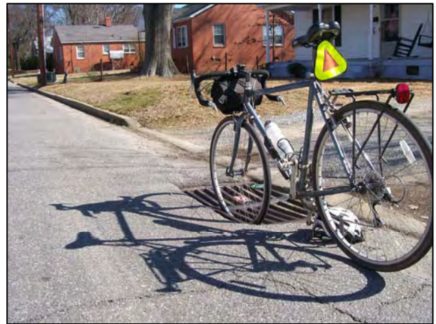
A “tire eater” on Church Street can cause injury
