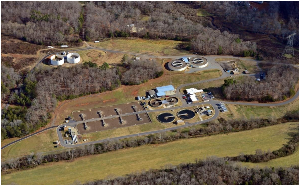
Rocky River Wastewater Treatment Plant
